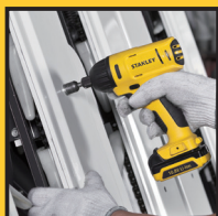
7 Driving Screw Into Window Frame 10.8V Impact Driver SCI12152
